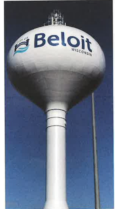
Beloit's I-90 Water Tower Picture by Jim Orr
